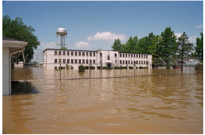
Renz Correctional Center's main administration/dormitory building during the Missouri River flood of 1993. The high water level caused the facility's permanent closure. Photo by Mark Schreiber, July 8, 1993 (MS297_251_096_04).
