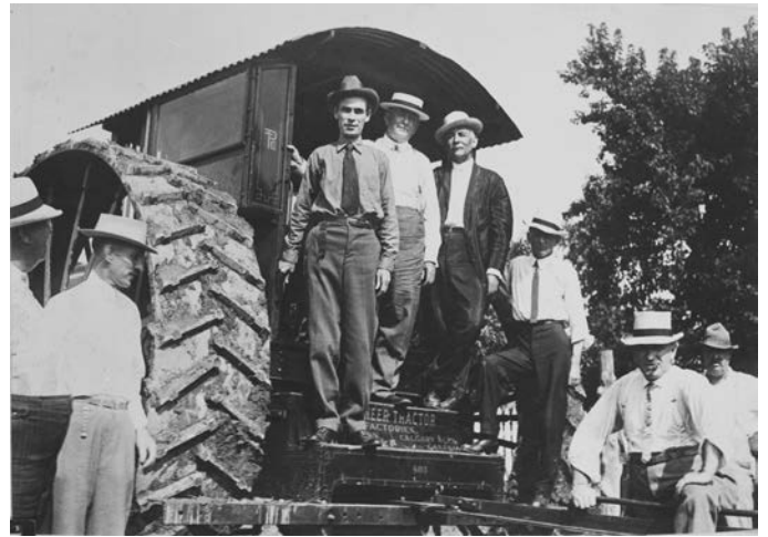
Gov. Major (left) on a steam powered tractor used to grade the road bed between Columbia and Jefferson City as part of the Governor's Good Roads Initiative. August 21, 1913.
