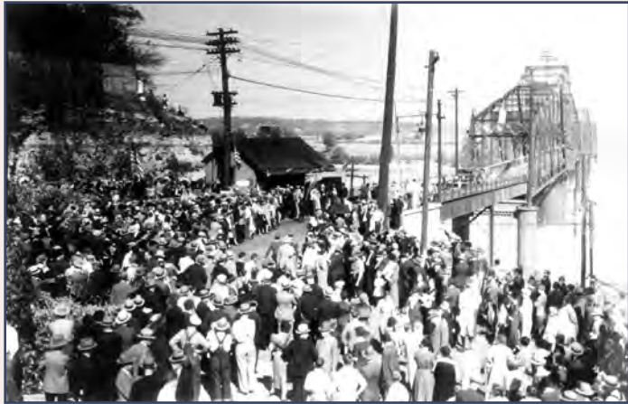
Last toll crossing on the 1896 bridge, October 15, 1932.
