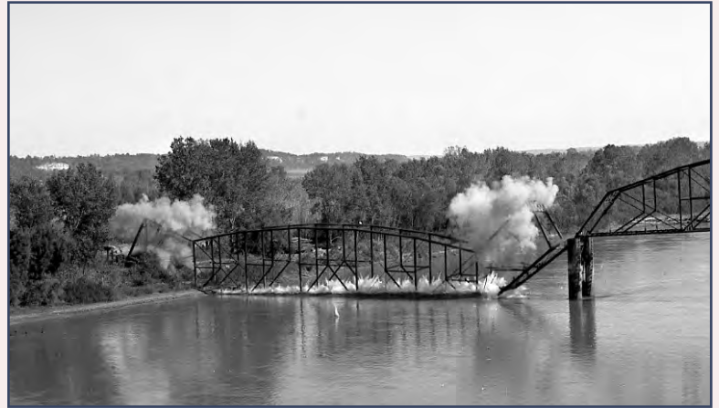
Demolition of the 1896 bridge, October 19, 1955.
