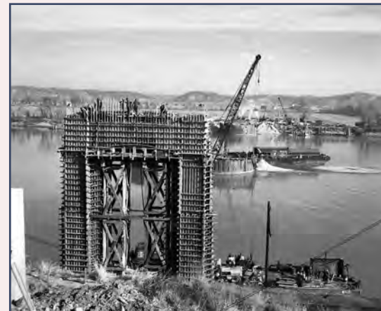
Pier construction for the new bridge, November 28, 1953.
